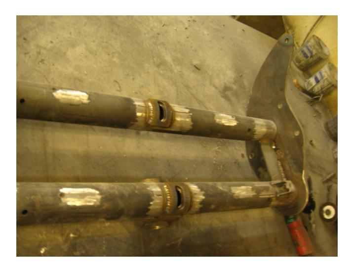
8) Drill two 1/2" holes 1" apart in the center of the beam. Be careful on what angle you position them at, as it wil limit your adjustablilty. Then, cut between the two hole so that you have a slot for the adjuster bolt to move in. Finally weld the adjuster plate to the beam tube, take your time welding so that the beam tube does not warp.
